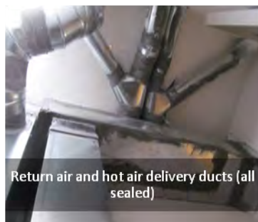
Geothermal (electric) heating system
