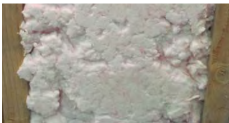
Fiberglass Blown In: R2-R.28 per inch Cost: $.70 to $2.00 per sq. ft. installed
