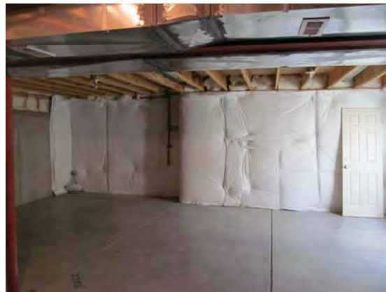
An insulated basement in a 5-year-old home.
