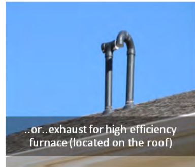
Exhaust for high efficiency furnace (located on the side of the house)
