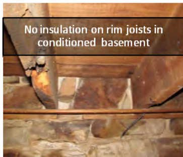
Water condensation in crawl space caused mushrooms to grow
