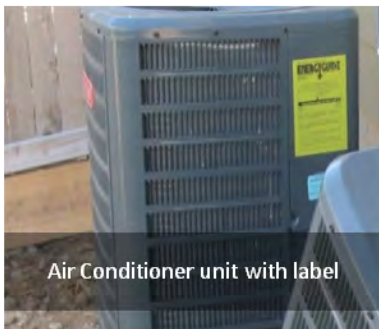
Close up photo of label on AC unit: 14 SEER
