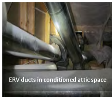
R8 insulation on ductwork in attic (to reduce noise from the ERV)
