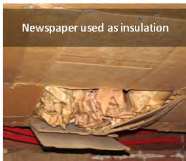
No insulation on rim joists in conditioned basement
